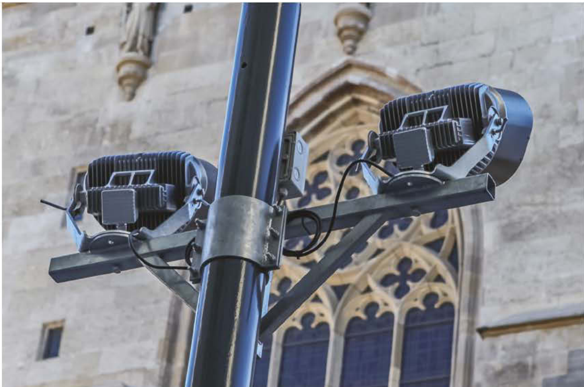
Mast - Montage LED Fluter FL200 - 190W - 4.000k
